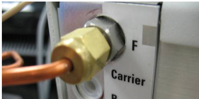
Figure 472. Plumbing the Nitrogen Supply to the GC
