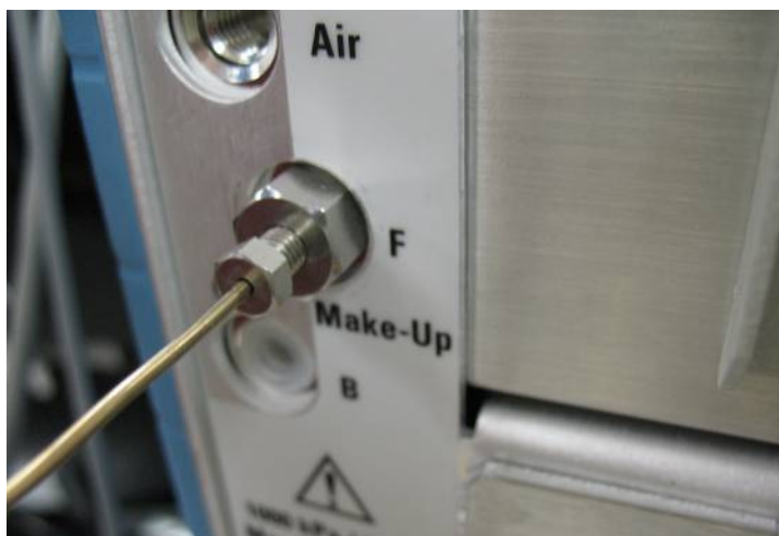
Figure 469. Plumbing the Helium Cylinder
