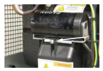
3. Remove the cover protecting the start components by placing a small flat head screwdriver into the center slot located at the bottom of the cover. Gently depress the tab (up or down?) until the catch releases. Pull the bottom out and up to remove
