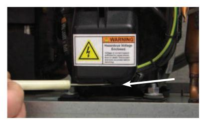
4. Mark the wires and there locations to assist with the rewiring of the condenser fan motor.
