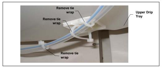
Figure 5-26. Removing Tie Wraps (Typical Installation Points)
