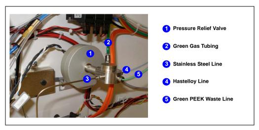
Figure 5-16. Connections to the Pressure Relief Valve
