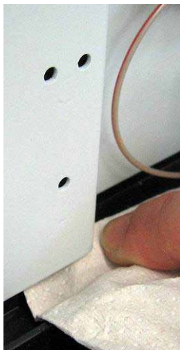
Fig. 40: Drying the leak sensor
