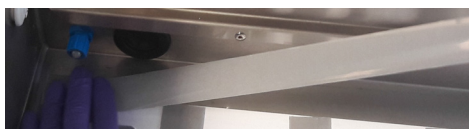
Figure 41. Apply upper sealing
