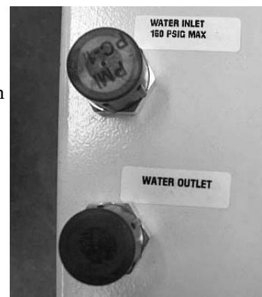
Figure 5-9. Inlet/Outlet Fittings
