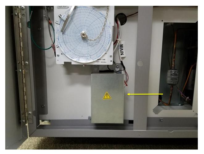
The battery(s) are located at the front of the compressor deck, behind the bottom front panel door. The yellow arrow is pointing to bracket that holds battery in place.
